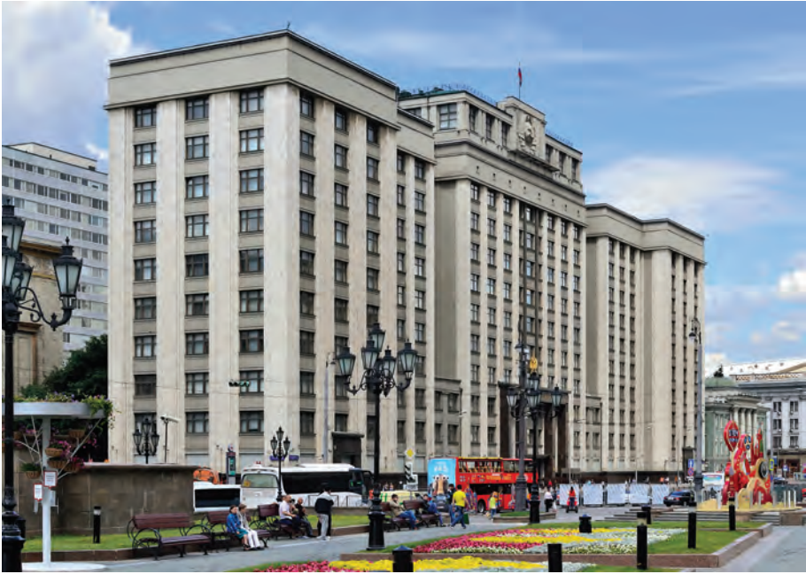
Figure 15.1 The current headquarters of the State Duma, adjacent to Manezh Square in the centre of Moscow. Architect: Arkady Langman. Originally built in 1932–1935 as the seat of the Council of Labour and Defence. © Dmitry Ivanov, 9 July 2016. Source: Wikimedia Commons, reproduced on the basis of a CC BY-SA 4.0 licence. Available at: https://commons.wikimedia.org/wiki/File:Building_of_Council_of_Labor_and_Defense,_Moscow.jpg (accessed 25 July 2023)
